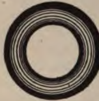
FIG. 67.—Rubber-ring for excluding auto-pulsations.
